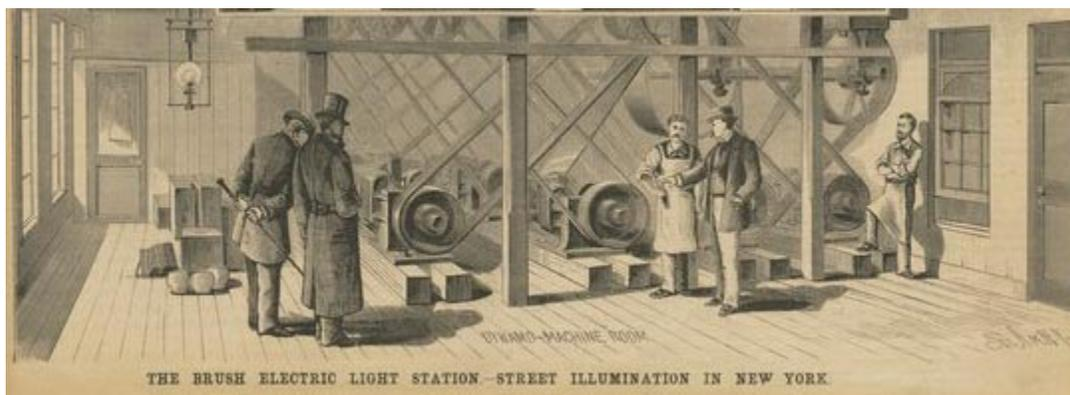
Source: Wikipedia. New York central power plant dynamos powered arc lamps for public lighting. Beginning operation in December 1880 at 133 West Twenty-Fifth Street, it powered a two mile long circuit.
